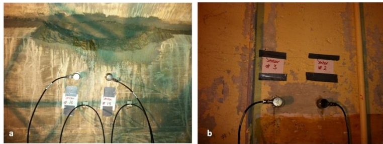
Figure 5.3 Photograph of: (a) horizontal beam location, and (b) control location.
